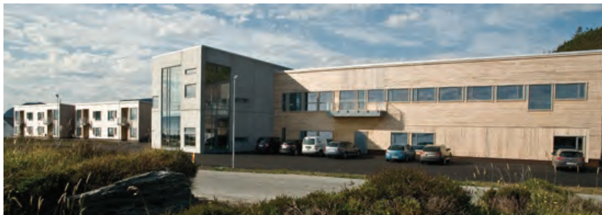
Figure 1. The Runde Environmental Centre main building, opened in 2009. REC is organized as a public-private shareholder company. See more information on http://www.rundecentre.no .
